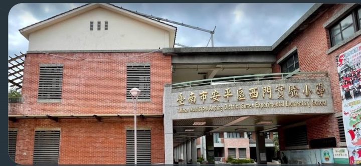
Simen Experimental Elementary School has experienced 5 floods
